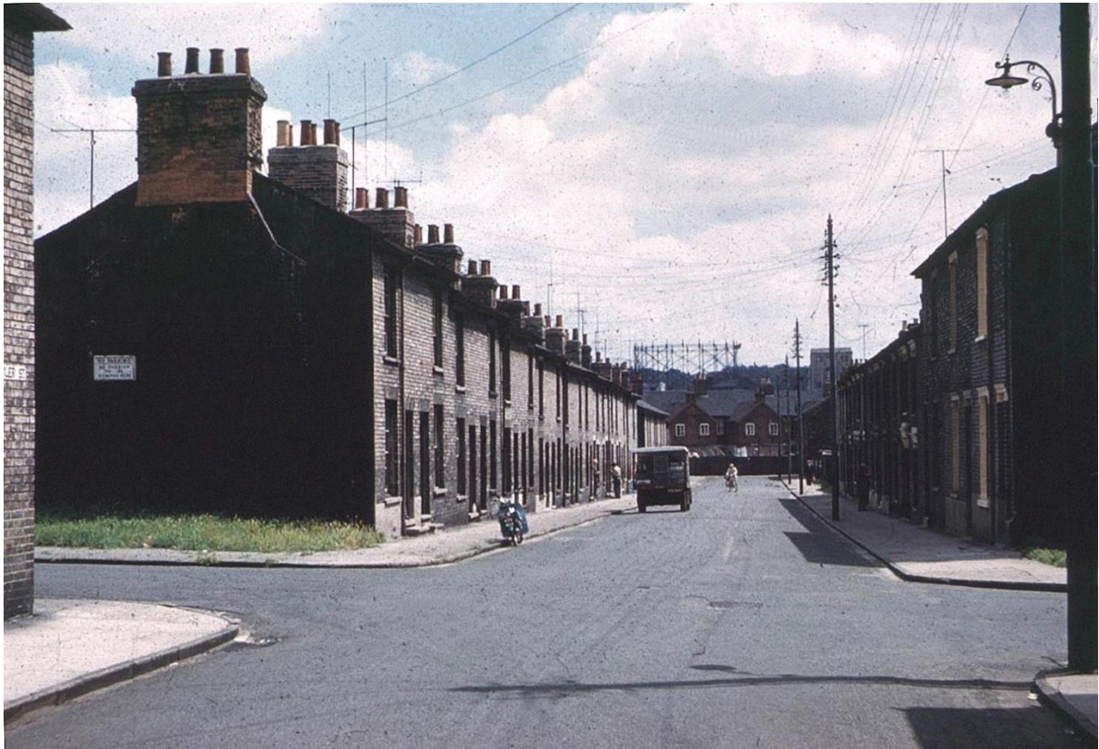
Lower Tyler Street at its junction with Hawes Street. IMT Image Archive Stuart Grimwade (ICBC) Collection
