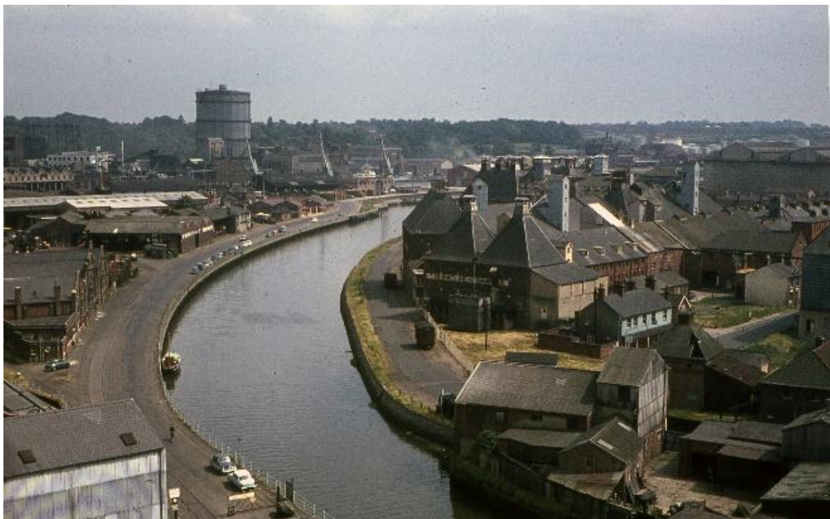
The Cut from Cranfield's Mill c.1970.
