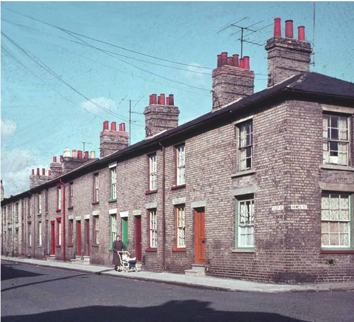
Upper Tyler Street at its junction with Hawes Street.
